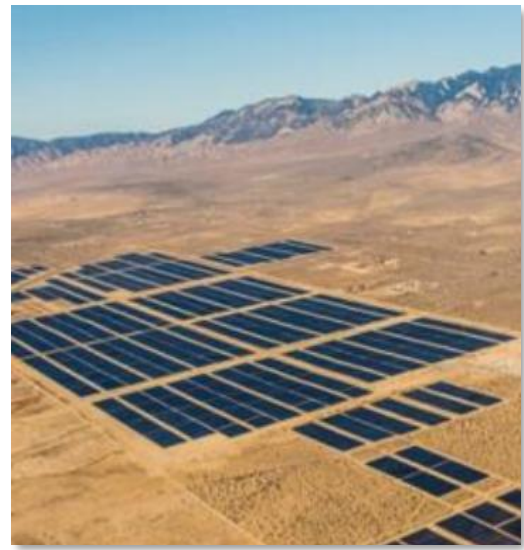
Lorax – a solar energy and battery storage infrastructure project in California, USA
